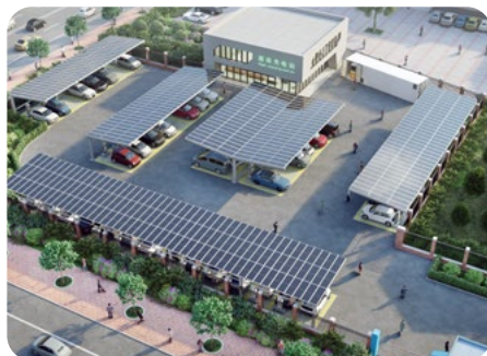
Solar-plus-storage and EV Charging Carport
